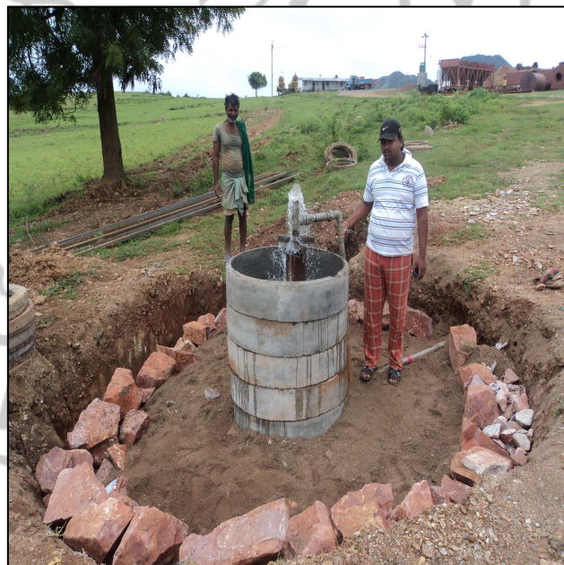
Figure 3.25: Rainwater recharge pit around the bore well
