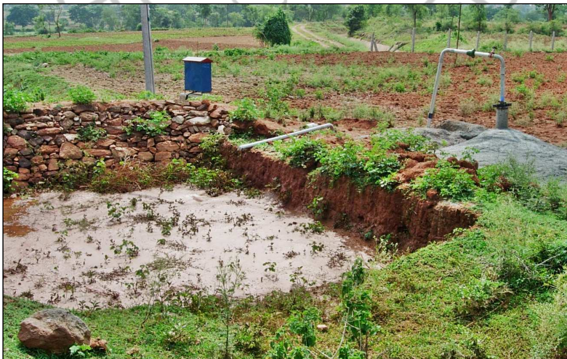
Figure 3.27: A stone check dam near for recharging a bore well
