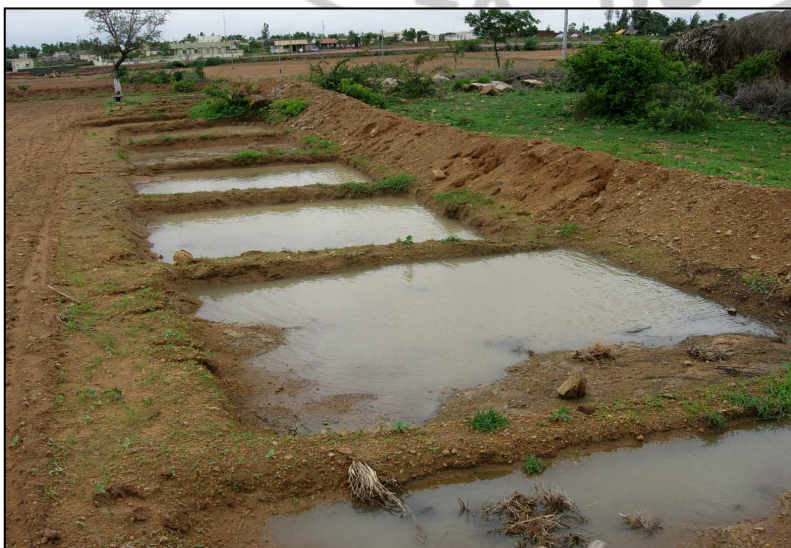
Figure 3.21: Runoff collection pits
