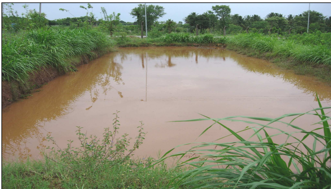
Figure 3.22: Deep pit for runoff collection and percolation
