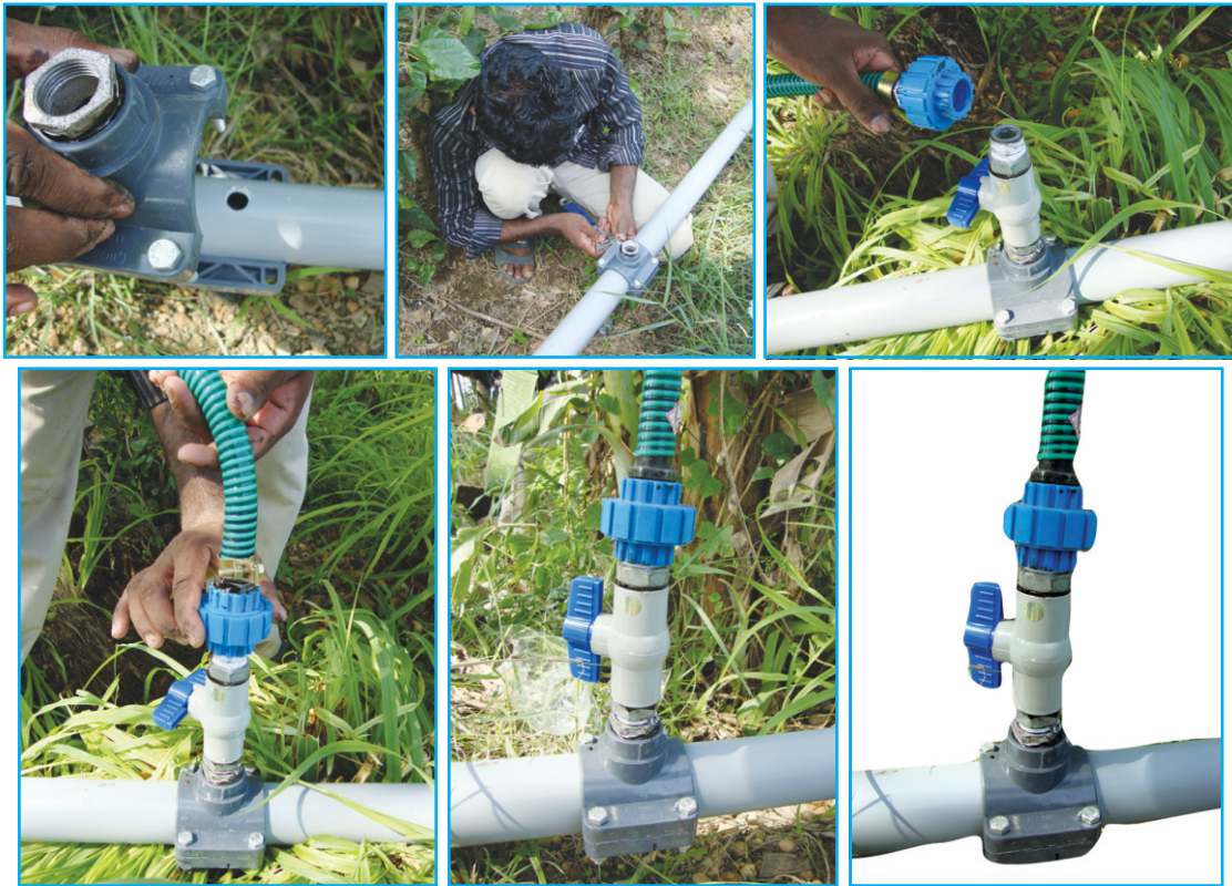
Steps involved in establishment of water jetting system in mulberry garden
