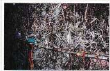
Silkworm rearing house walls made of bamboo leaves
