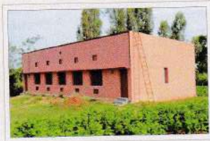
Gable end roof
