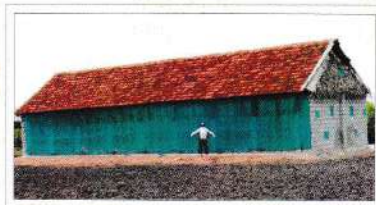
Silkworm rearing house walls made of bamboo leaves
