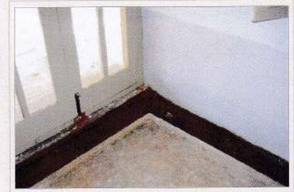
A water channel all around the silkworm rearing hall
