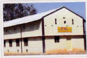
Lean to wall roof
